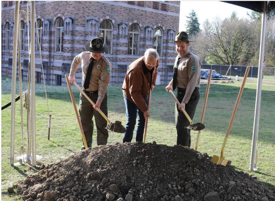
Kevin Daniels of Daniels Real Estate helps state park rangers shovel dirt at the ceremonial groundbreaking for the Lodge at Saint Edward Park on Dec. 7. His company is restoring and renovating the seminary building in the park. Katie Metzger/staff photo
